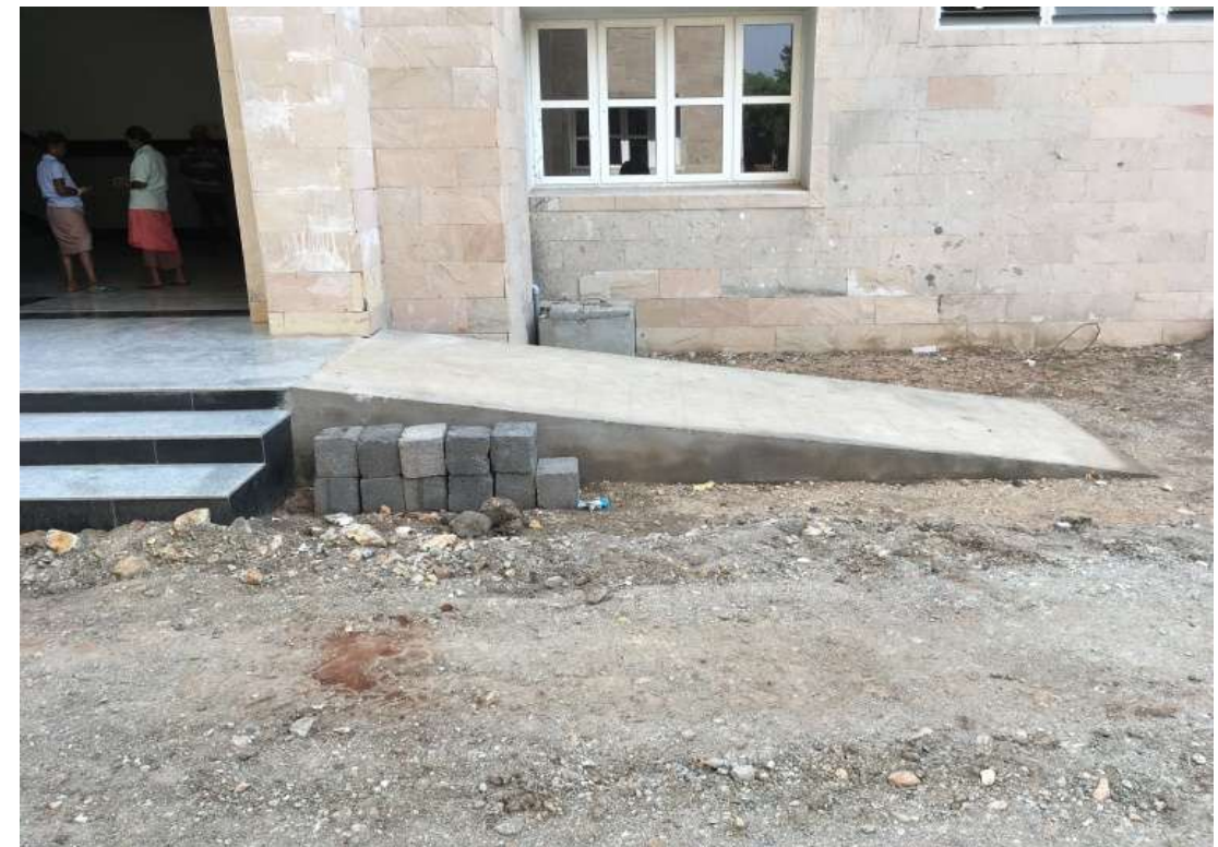
PROVISION OF RAMP FOR THE DISABLED PERSON TO ACCESS THE BUILDING.
