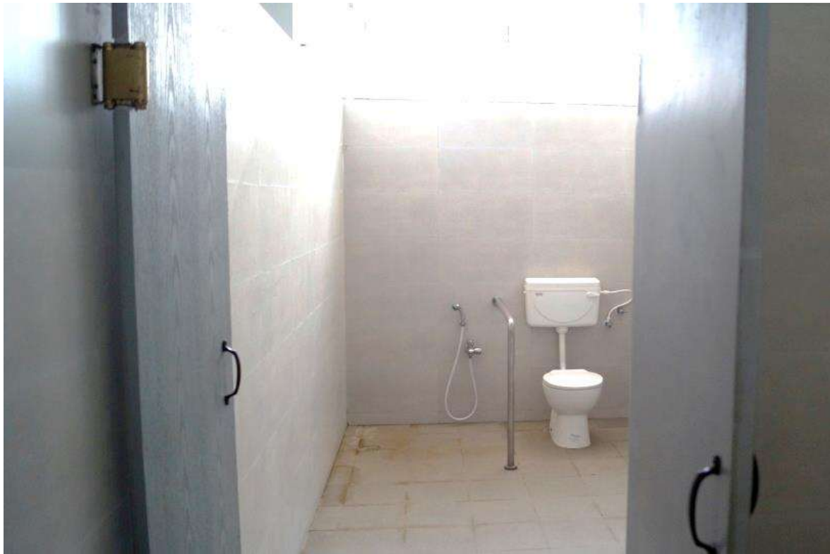
PROVISION OF DUAL SWING OPERABLE DUAL DOOR SHUTTERS PROVISION OF GRAB BARS FOR THE DISABLED TOILET.
