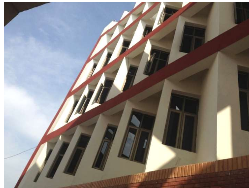
Louvers acts as passive sustainable elements protecting the interiors from heat
