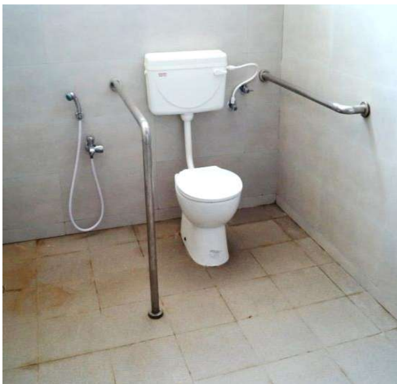
PROVISION OF DUAL SWING OPERABLE DUAL DOOR SHUTTERS PROVISION OF GRAB BARS FOR THE DISABLED TOILET.
