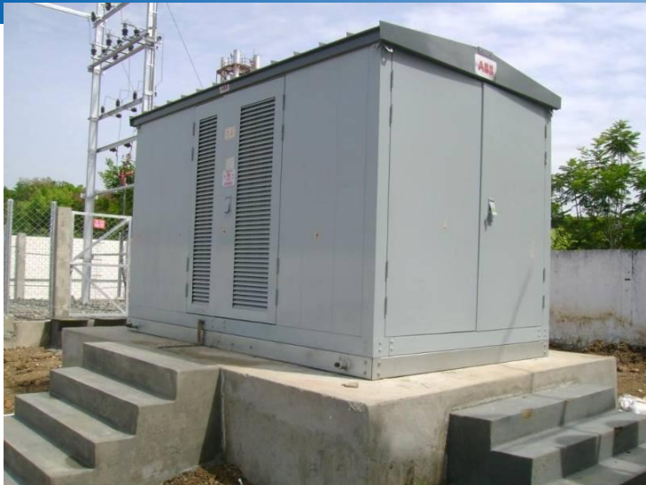
Compact Substation (CSS)
