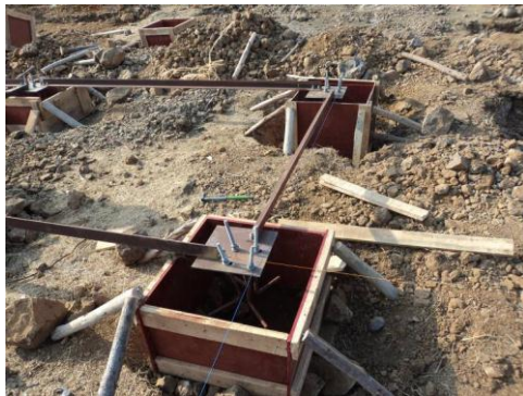
Templates for Foundations
