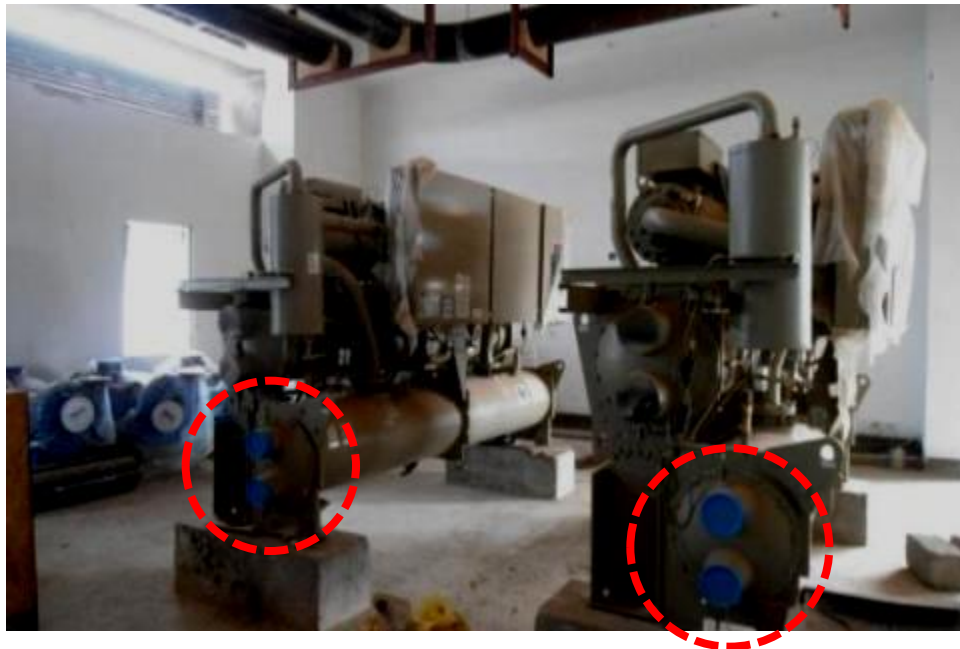
Protection of MEP Equipments, Materials etc. Being procured at site
