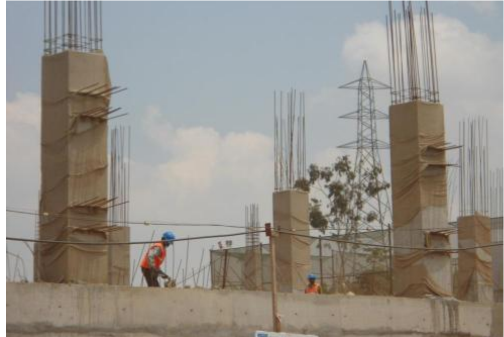
Use of Gunny Bags and Treated Grey Water for Curing Purpose
