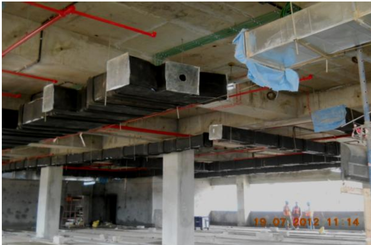
Covering the loose ends of the ductwork presently ongoing
