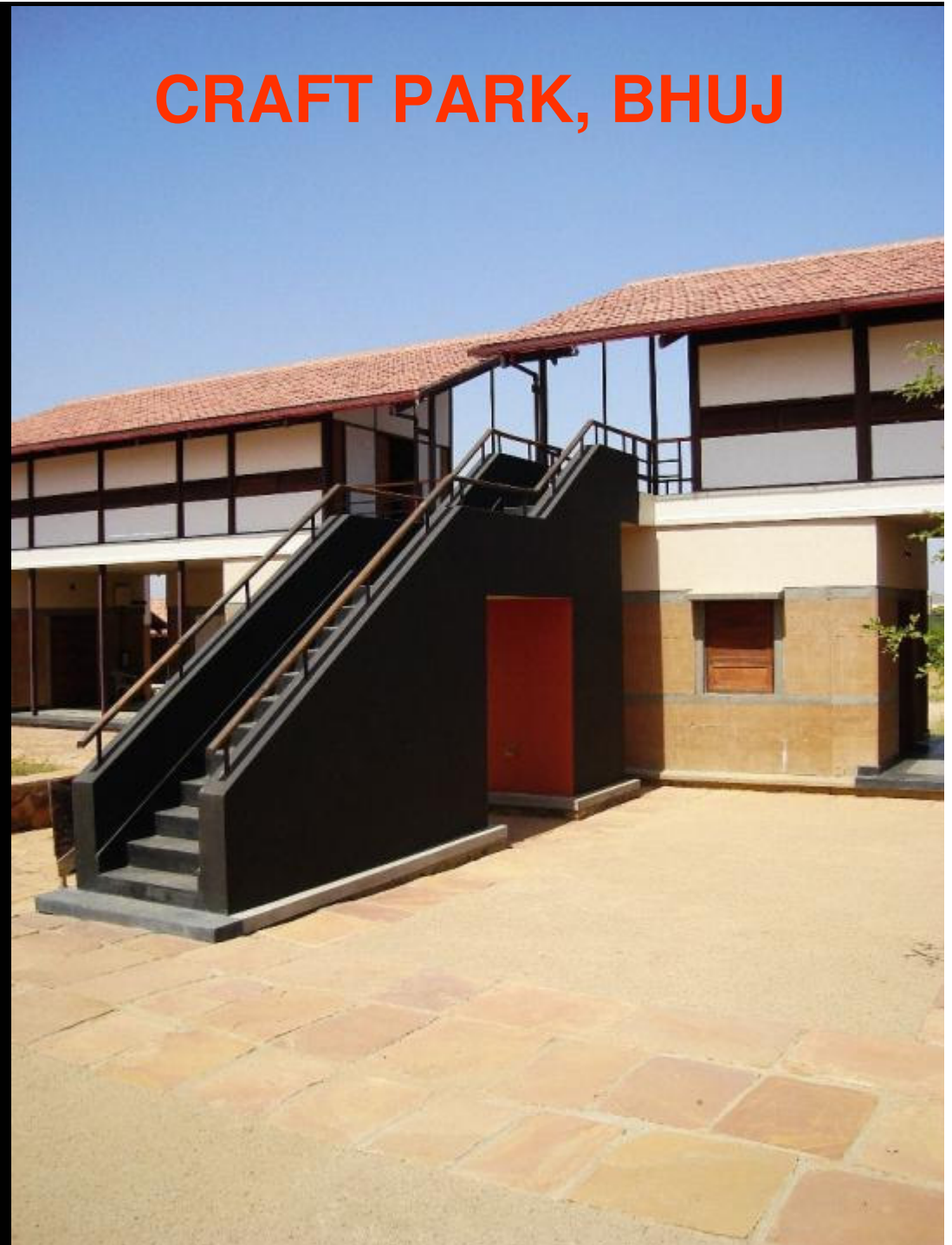
Weight reducing vertically: Stone - rammed Earth - soil blocks - wattle and daub.
