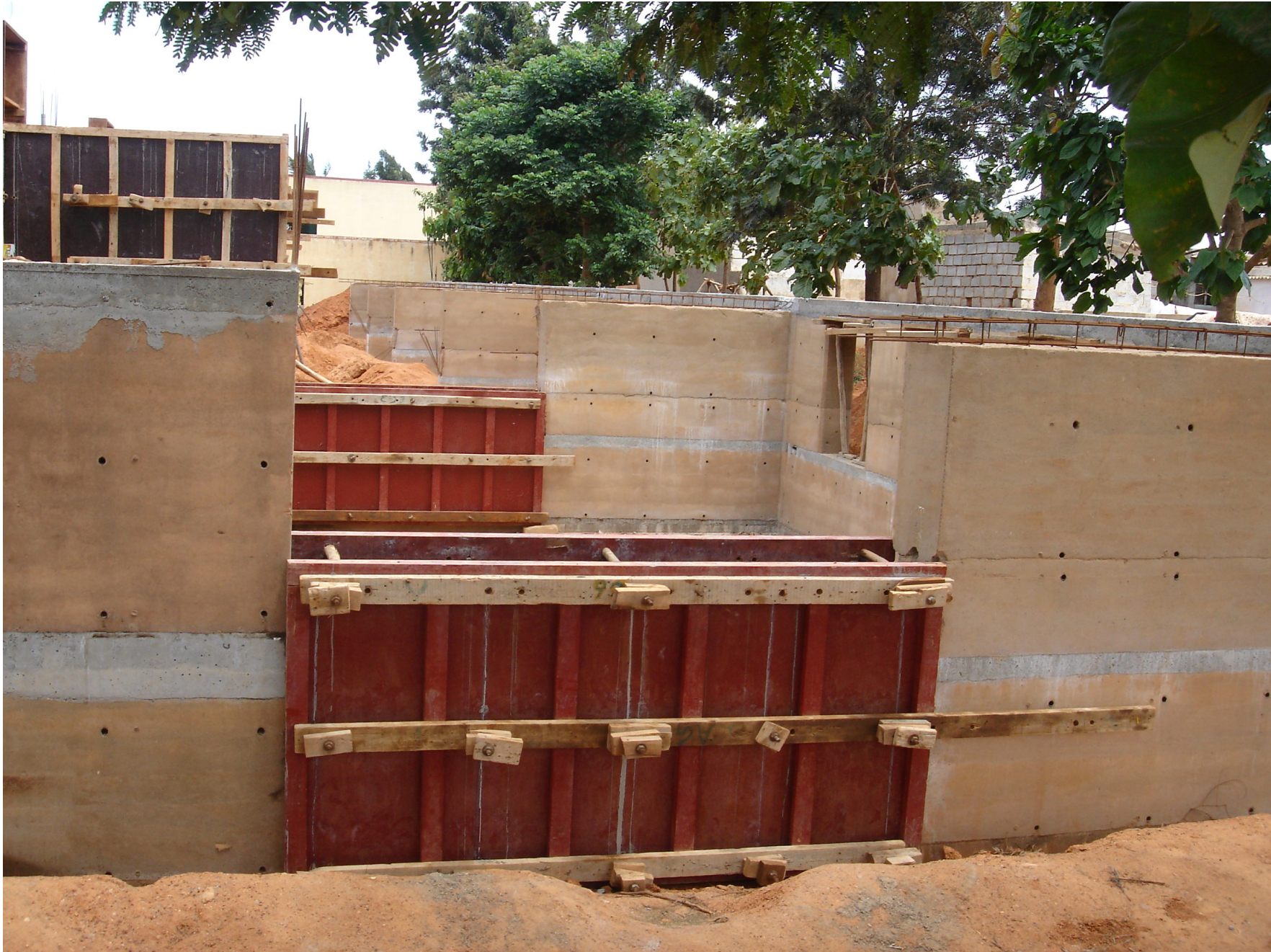
CSRE walls under construction – 3 storey buildings
