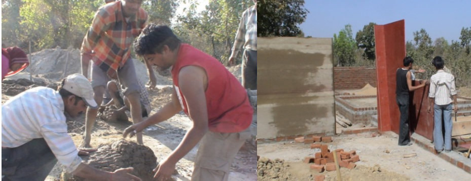
Cob And Rammed Earth walls, using/developing using local skills
