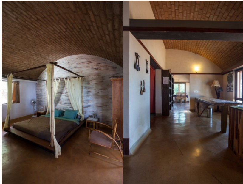
INTERIOR -MANAGER'S BUNGALOW..BRICK VAULT CEILINGS
