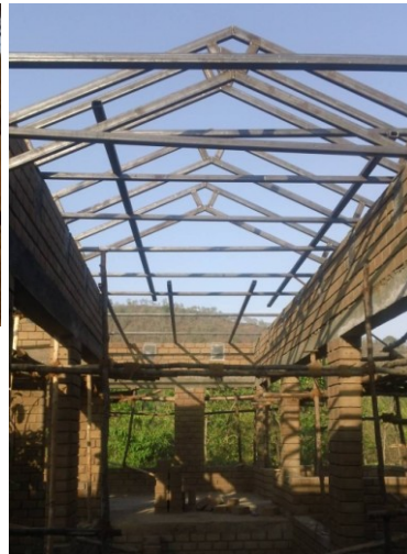
BED BLOCKS CONNECTED WITH ROOF BAND
