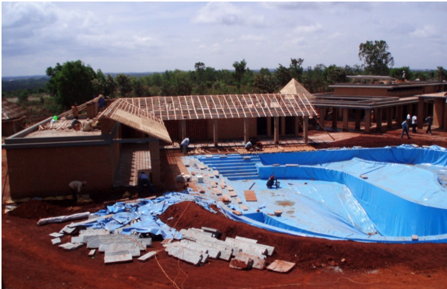
BIO-POOL DURING CONSTRUCTION
