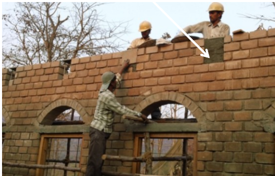
BED BLOCKS CONNECTED WITH ROOF BAND
