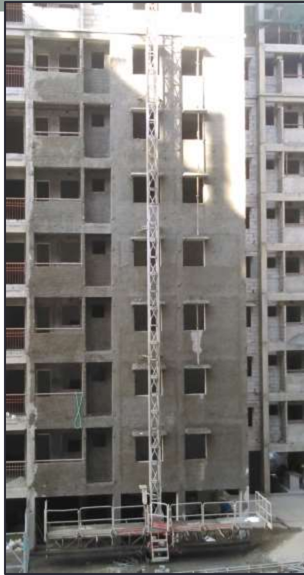
VIEW OF EXTERNAL PLASTERING IN PROGRESS..
