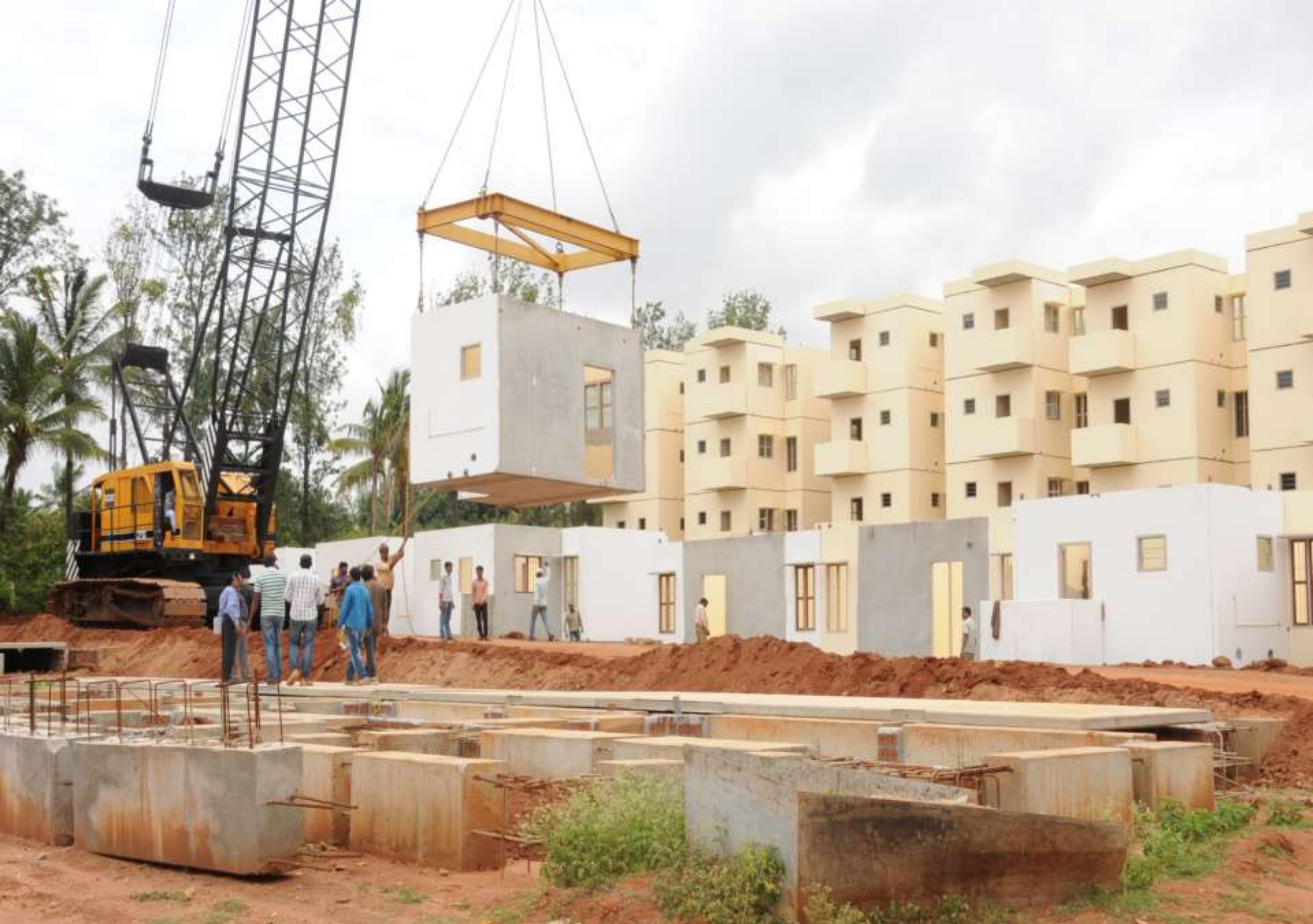
Placing of Housing Units
