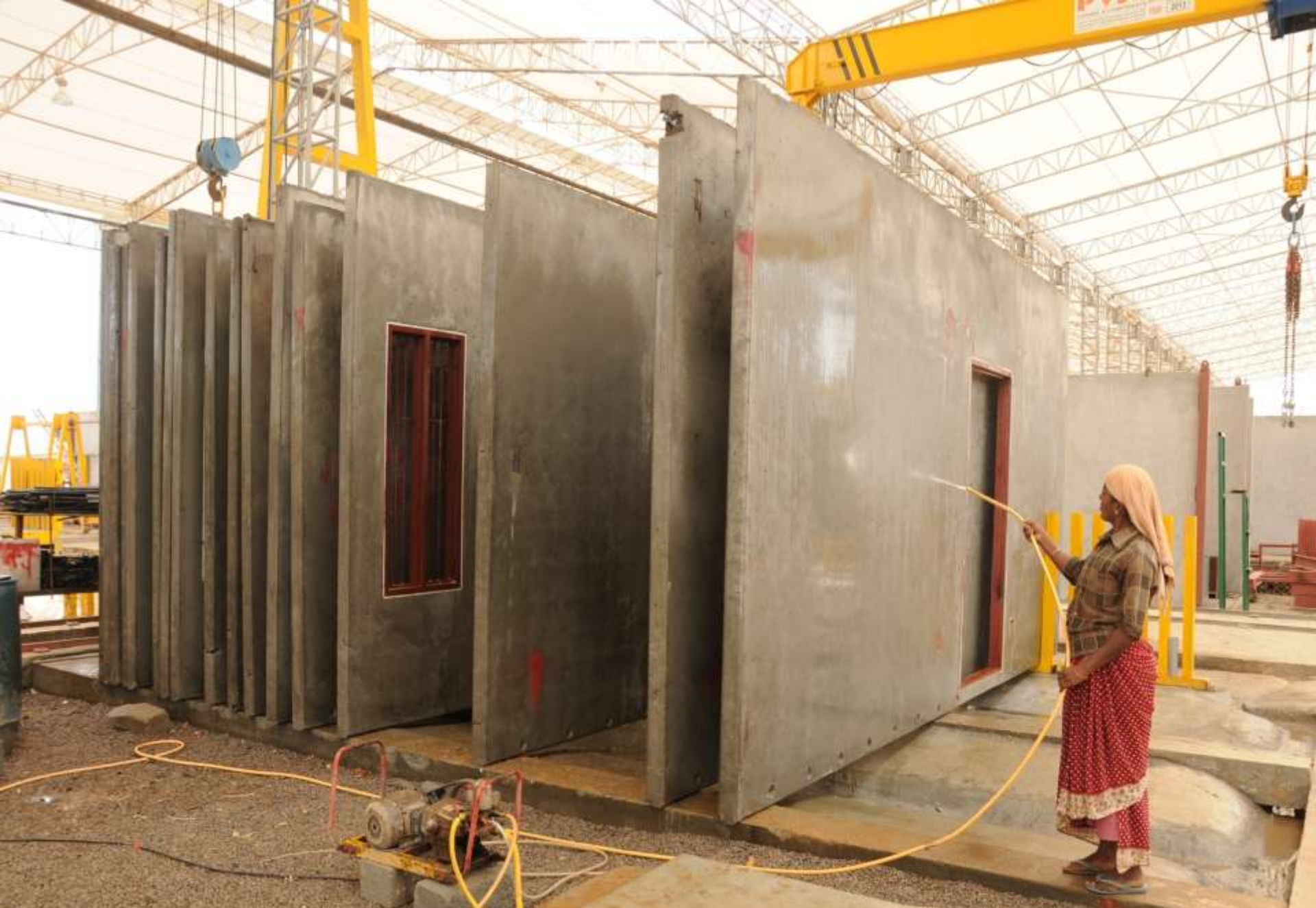
Hardened Concrete Panels
