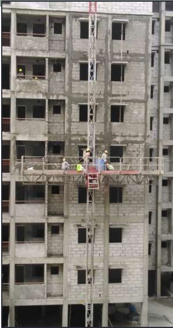
VIEW OF EXTERNAL PLASTERING IN PROGRESS..
