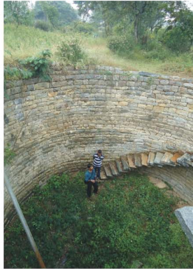
Large, dry open well adjacent to the site boundary now used through a bore-well
