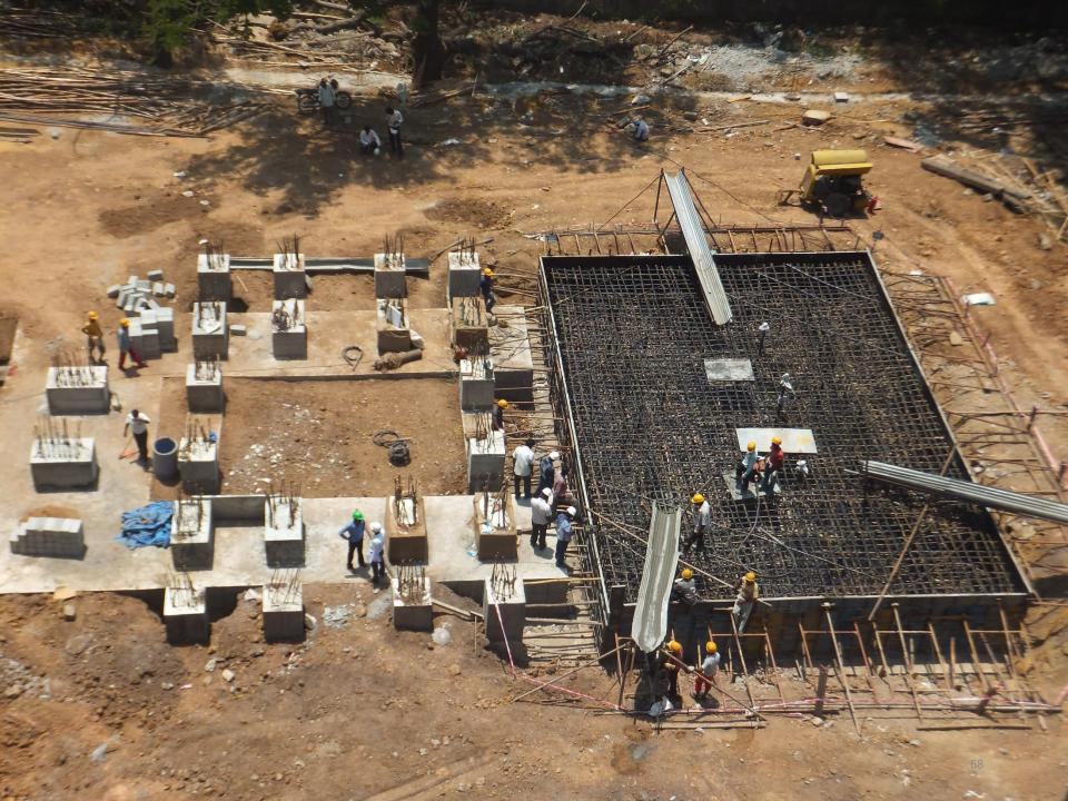
THUS BAMBOO CAN BE EFFECTIVELY USED AS **REPLACEMENT OF REINFORCING STEEL TO SAVE** • ENERGY. IN THE PROJECT OF JAIN TEMPLE, THE USE OF **• REINFORCING STEEL WAS NOT ALLOWED FROM** RELIGIOUS CONSIDERATIONS. SO BAMBOO WAS **USED IN PILE, PULE CAP, COLUMNS & BEAMS.** MORE WORK IS REQUIRED TO BE CARRIED OUT IN THIS FIELD.
