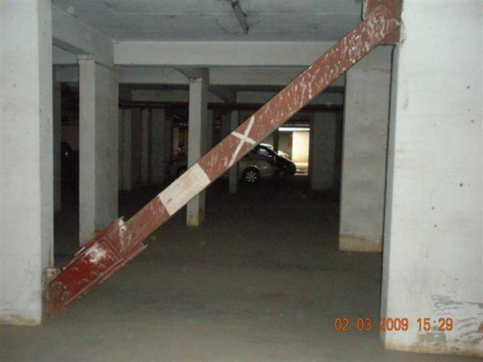
**USE OF FRICTION DEMPER REDUCE REINFORCING** SINCE THEY ARE STEEL BY 20% **NOW** MANUFACTURING IN INDIA WITH CANADIAN **COLLABORATION. THEY RESULT IN ECONOMY. NORMAL STRUCTURE DESIGN CATERS FOR 10% OF** MAXIMUM CONSIDERED EARTHQUAKE (MCE) BUT WITH USE OF FRICTION DAMPERS WE CATER FOR 130% OF MCE.
