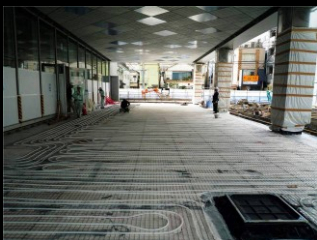
Open-air Floor Heating &amp; Cooling side of GSHP
