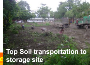
Top 200mm top soil removal from site
