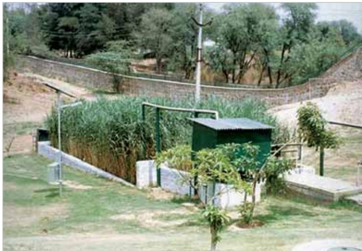
**Figure 7** Root zone system for waste water treatment
