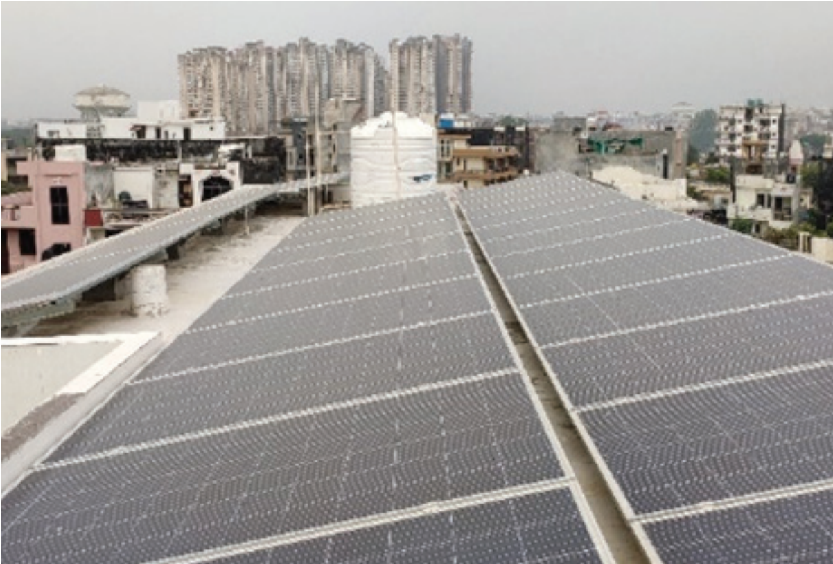
Image 8: Solar PV (10kW) installed on the rooftop
