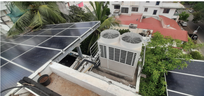
Image 4: VRV-based air conditioner with R410A eco-friendly refrigerant
