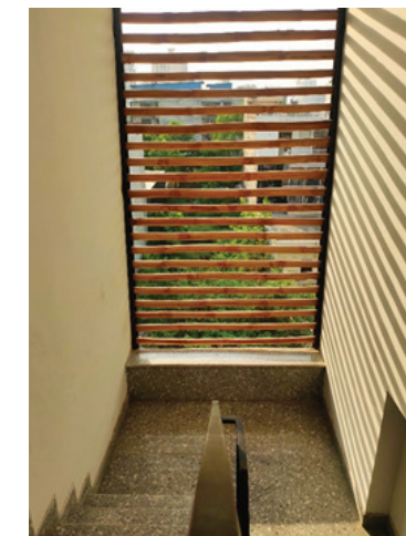
Image 2: Bamboo screen allows light and ventilation in non-habitable area
