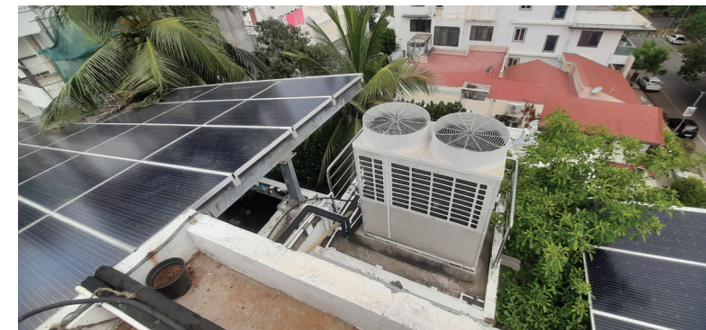
Image 2: Solar panel which acts as a roof for dining and break-out space
