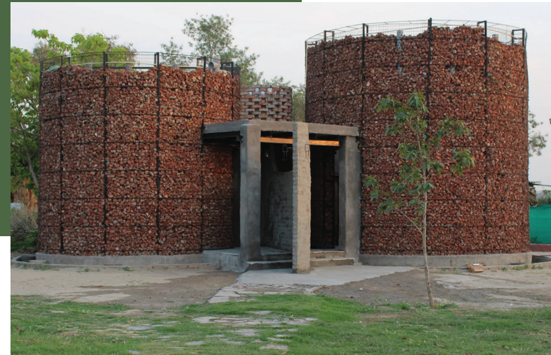
Image 3: Ant Studio's Twin Toilets in Noida, with CoolAnt Terrabyte (a gabion wall filled with damaged terracotta pots and other construction debris)
