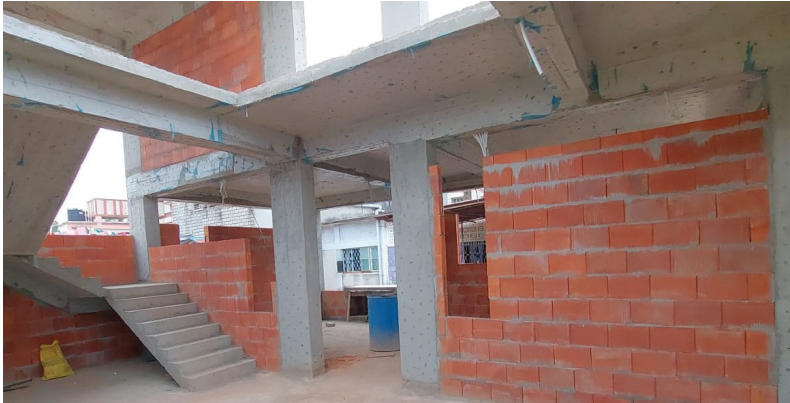
Image 5: House construction with hollow blocks
