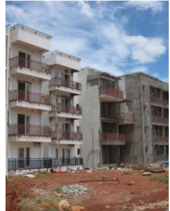
2012: Construction of EE homes in Bangalore
