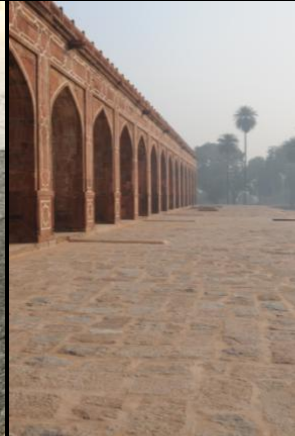
Lower Plinth restored in 2009
