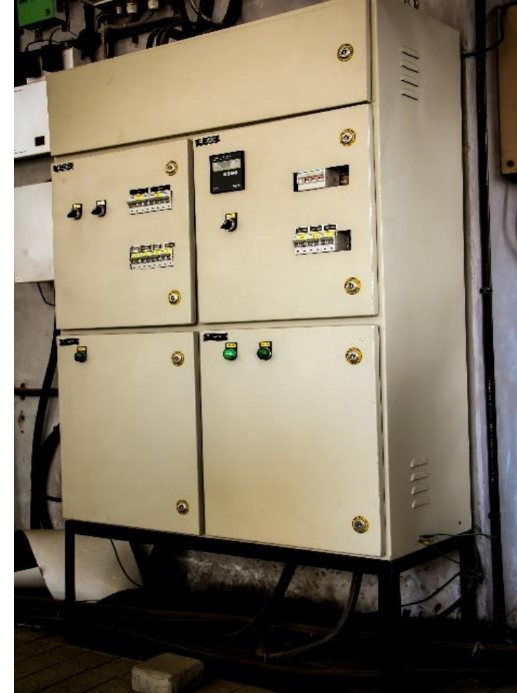
Automatic Transfer Switch
