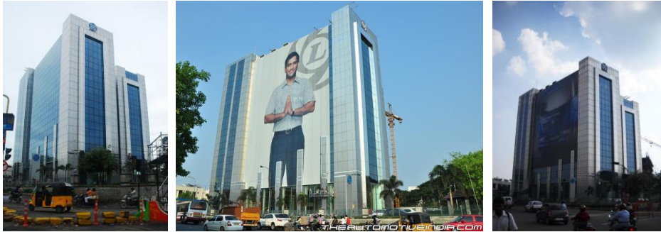
Ashok Leyland Office (West Façade), Chennai
