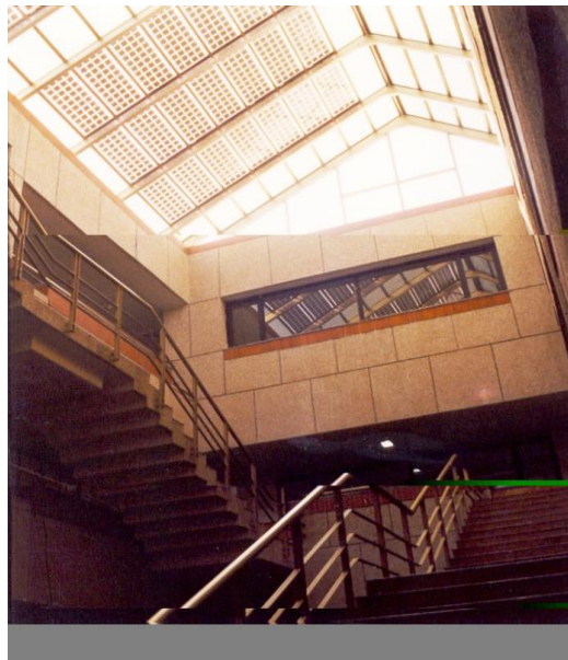
Daylight harvesting: BSBE Building, Kanpur
