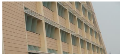
Light shelves allow daylight to penetrate deeper into the buildings
