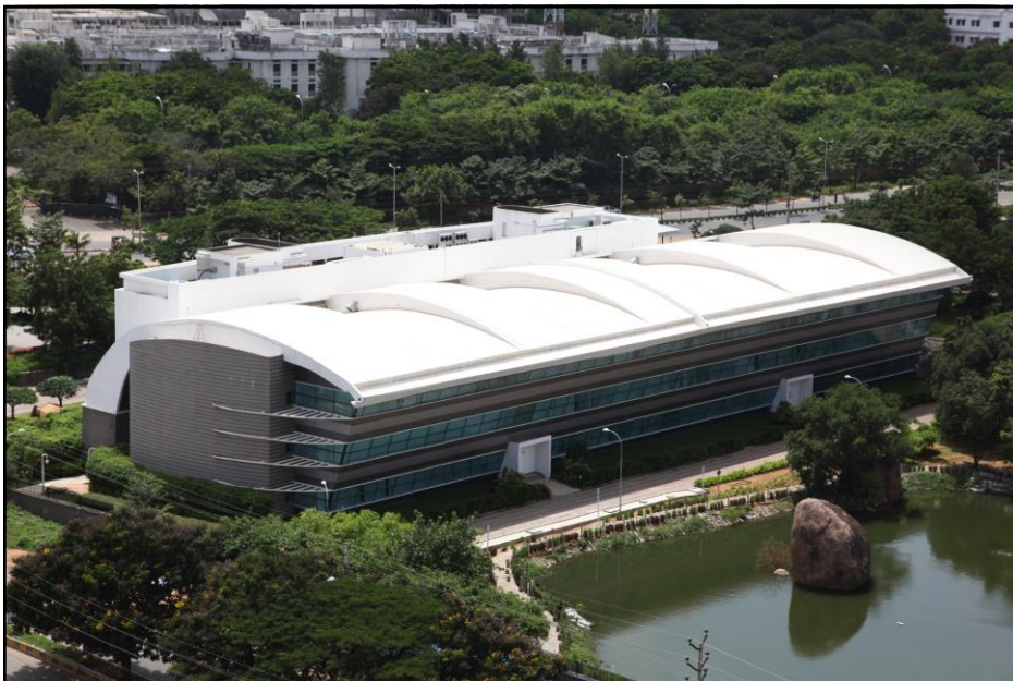
North Façade...has the maximum glazing
