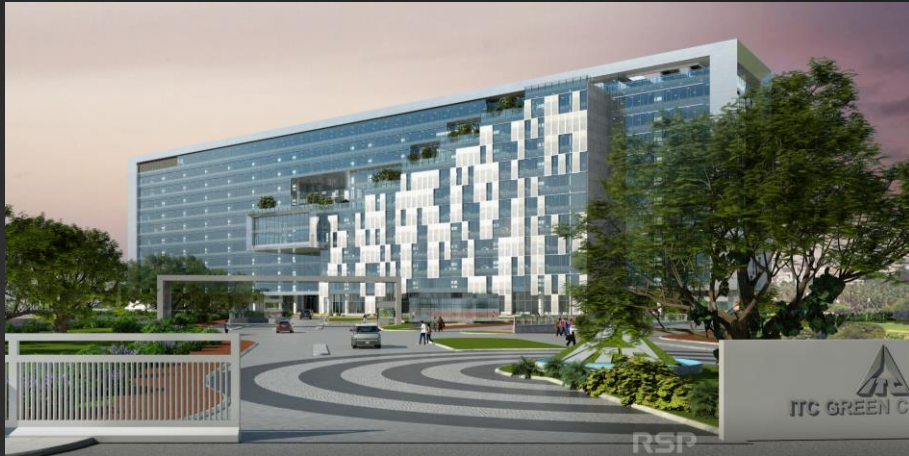
External (North &amp; South) Facade
