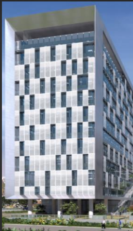
East and West Facade
