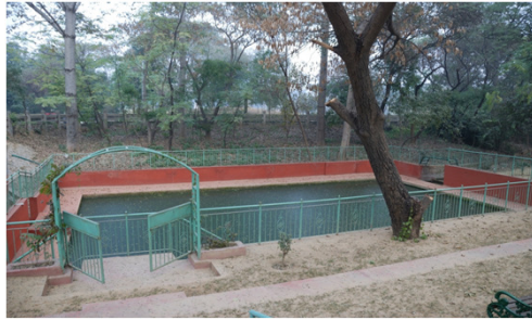
Water management plan for TERI-Gram campus - construction of artificial recharge injection wells; Rejuvenation of streams; Rainwater harvesting
