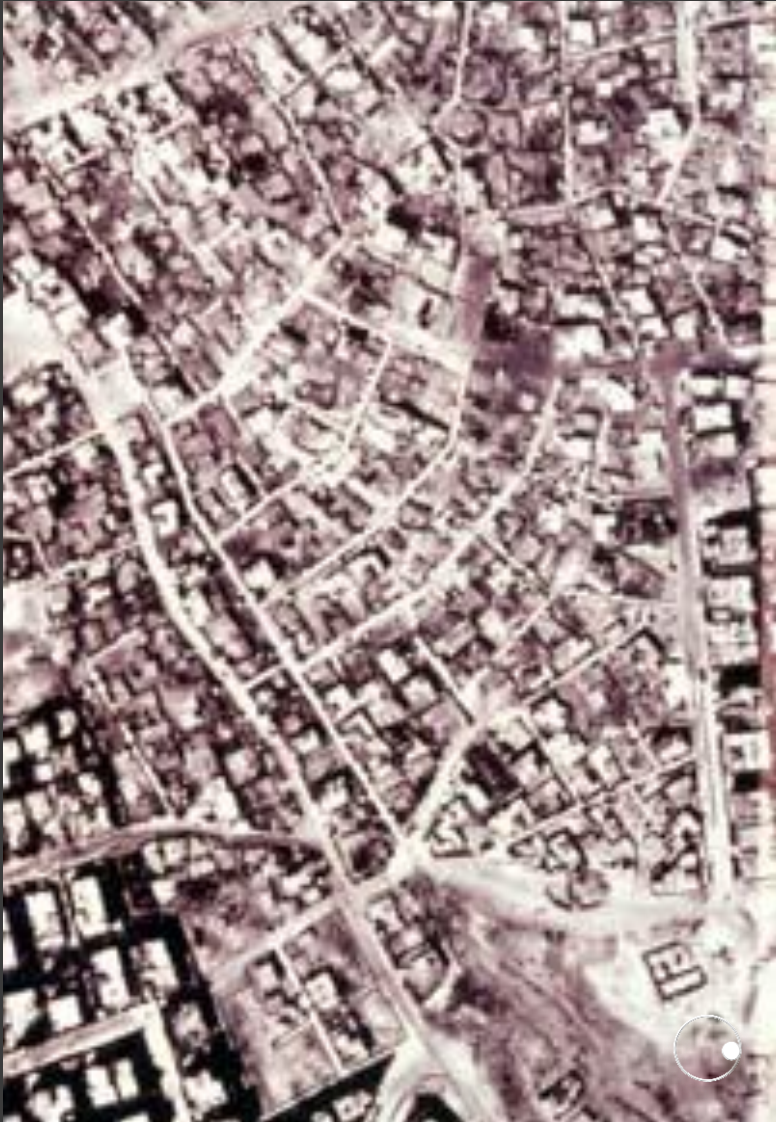
East Wahdat Upgrading Program, Amman, 1980s Source: Client Report, Aga Khan Award for Architecture
