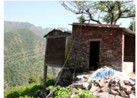
(c) Brick construction on stilts near Byasi
