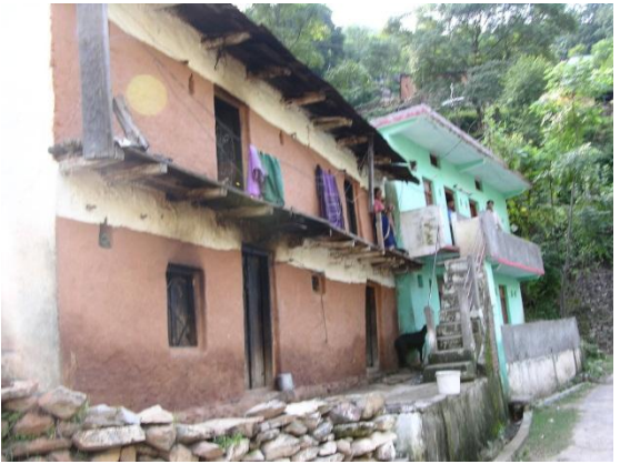
Random rubble stone masonry with mud plaster
