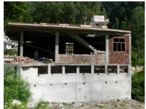
(b) Brick wall with RC frame in Tapowan
