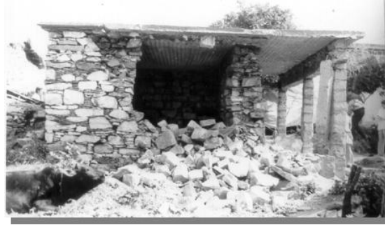
Damage to random rubble stone masonry During Chamoli Earthquake
