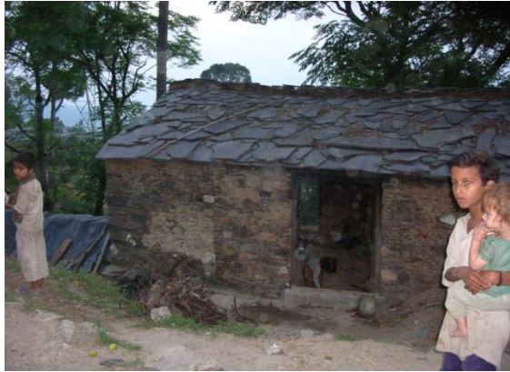
Slate Roof of a house in village Tamiyar
