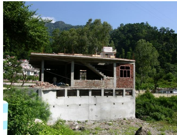
RCC Roofs of a residential building at Tapowan
