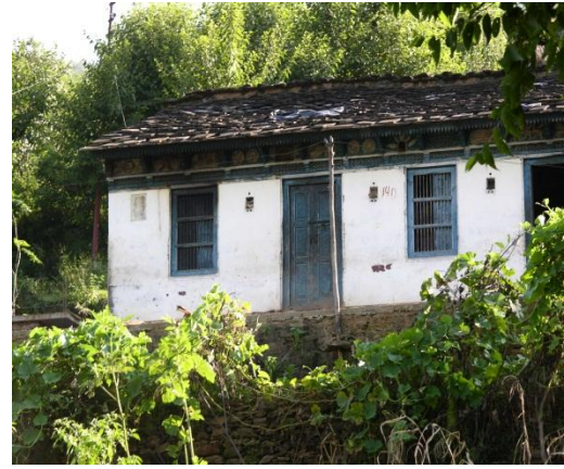
Random rubble stone masonry with cement plaster
