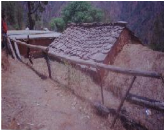
Mixed Roofs in village Pasar
