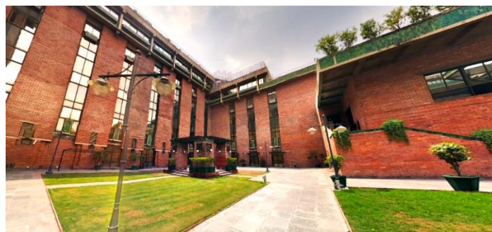
Plan and view of Char Minar in India Habitat Centre, New Delhi
