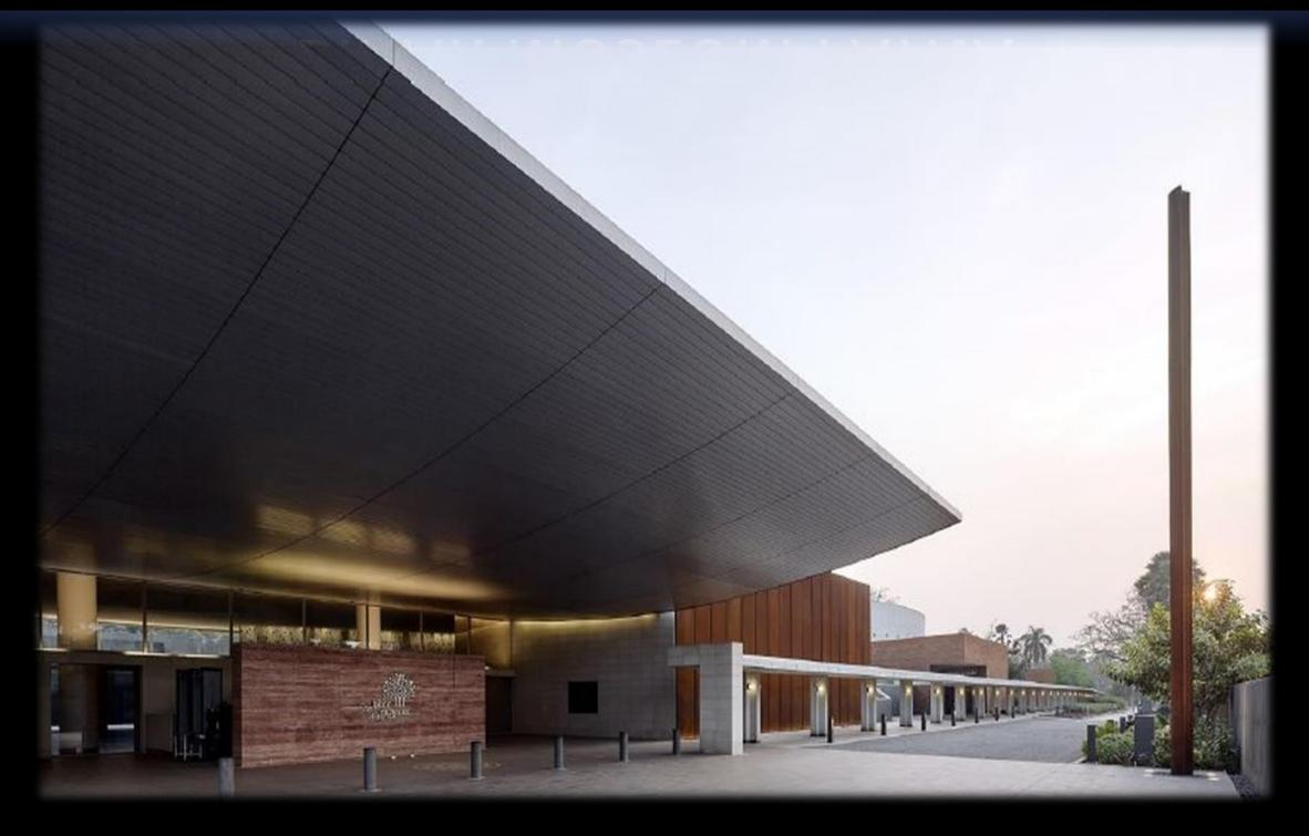
Favorable orientation to maximizes daylight and ventilation • Well-shaded fenestrations with overhangs, louvers and jaalis Optimized Window Wall Ratio i.e. 12% • Well-daylit Regularly occupied spaces
