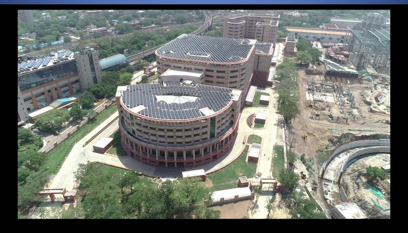
• Total installed capacity of Solar energy -1.47 MW • One of the largest installation with Solar PV panels on Institutional building in NCR region • 100% of renewable energy system to offset the energy consumption for internal artificial lighting
