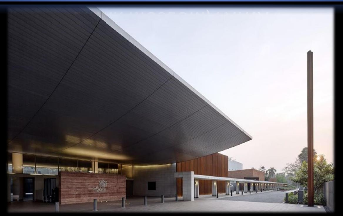
Use of fly-ash bricks for cavity wall construction • Use of flat slab technique • Embodied energy reduction of 35%
