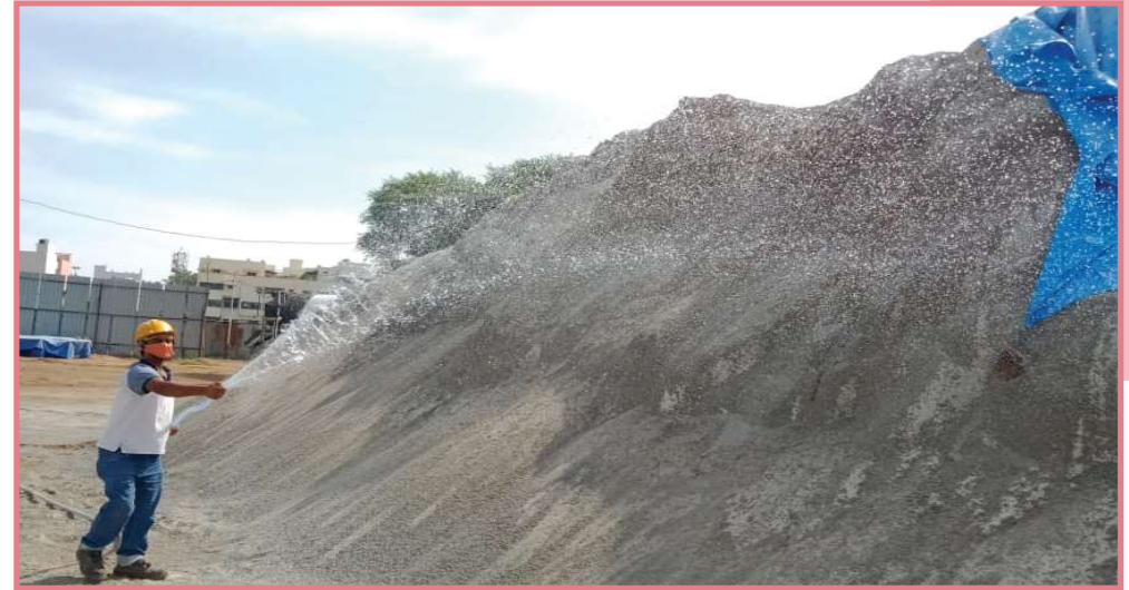
▲ Fine material being sprayed on with water by a worker
