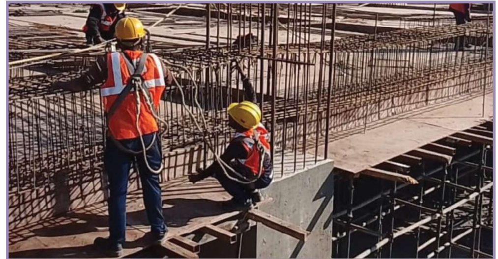
▲ Adherence of workers with safety harnesses working at height on-site.
