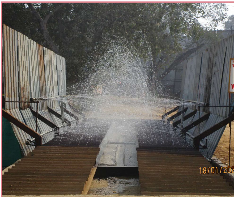
▲ Mechanical washing of tyres using sprinklers. The water is collected and reused again for washing.
