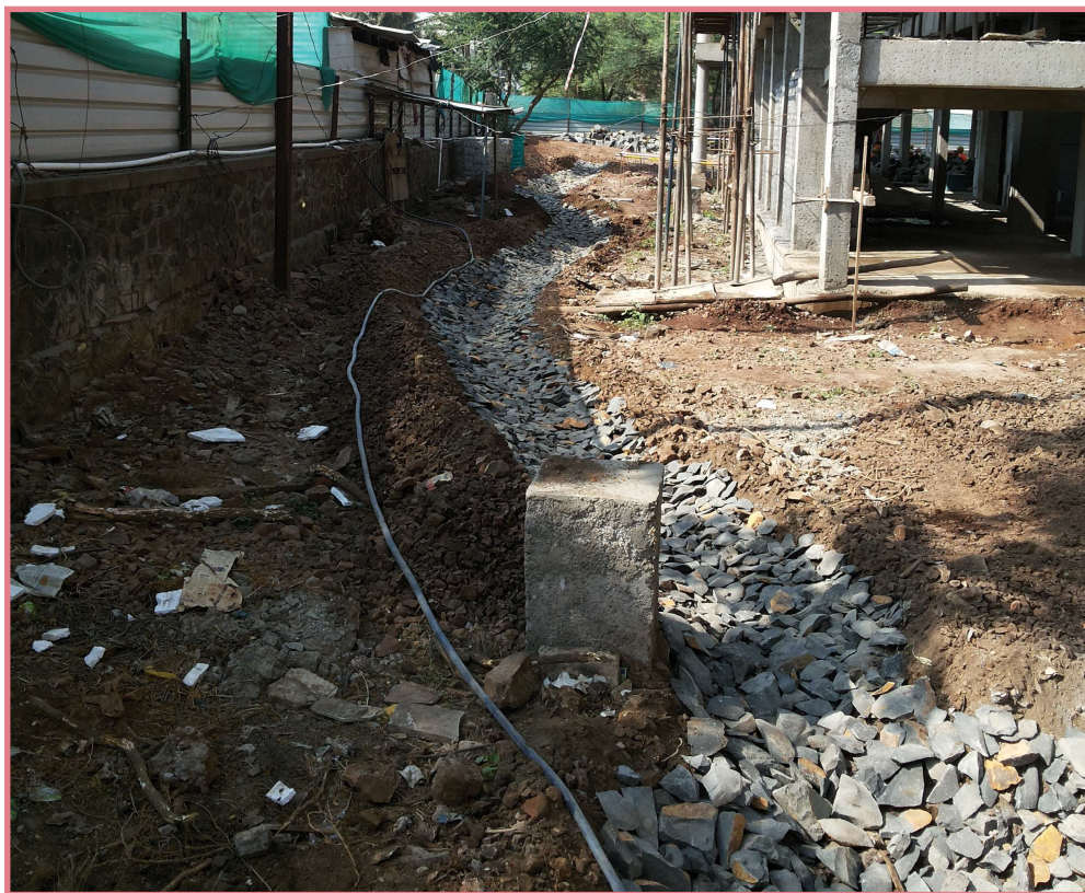
▲ Soil erosion channel with gravel bed
