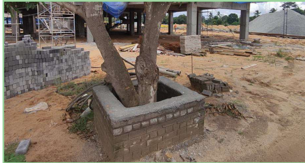
▲ Demonstration of barricading of trees using concrete blocks
