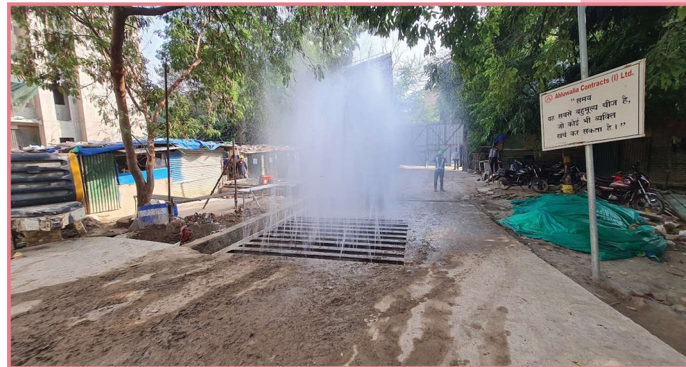
▲ Wheel-washing facility at the exit of the site
