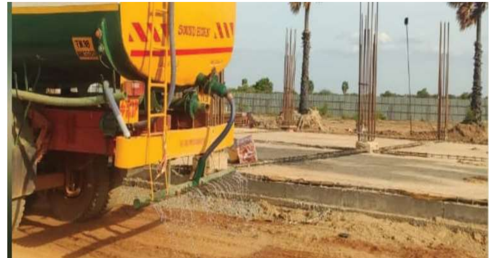
▲ Periodic water sprinkling of the road
