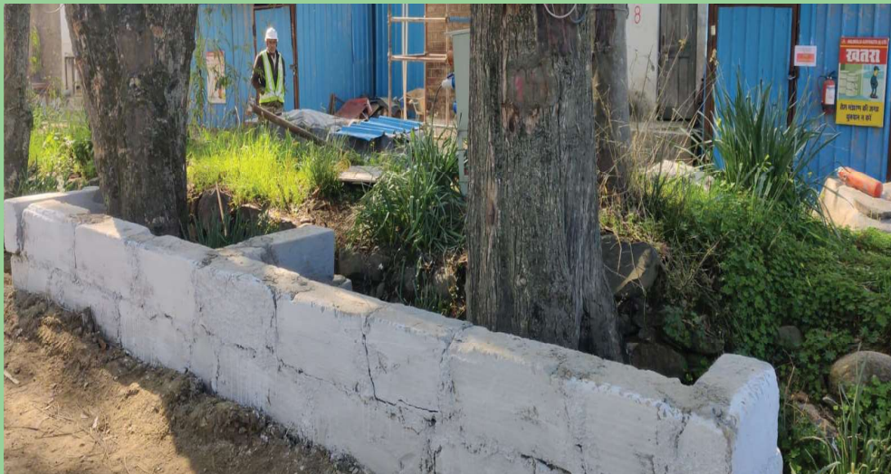
▲ Demonstration of reuse of waste concrete blocks to safeguard trees
