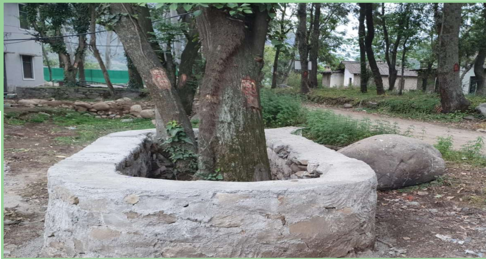
▲ Demonstration of barricading of trees using rubble masonry
