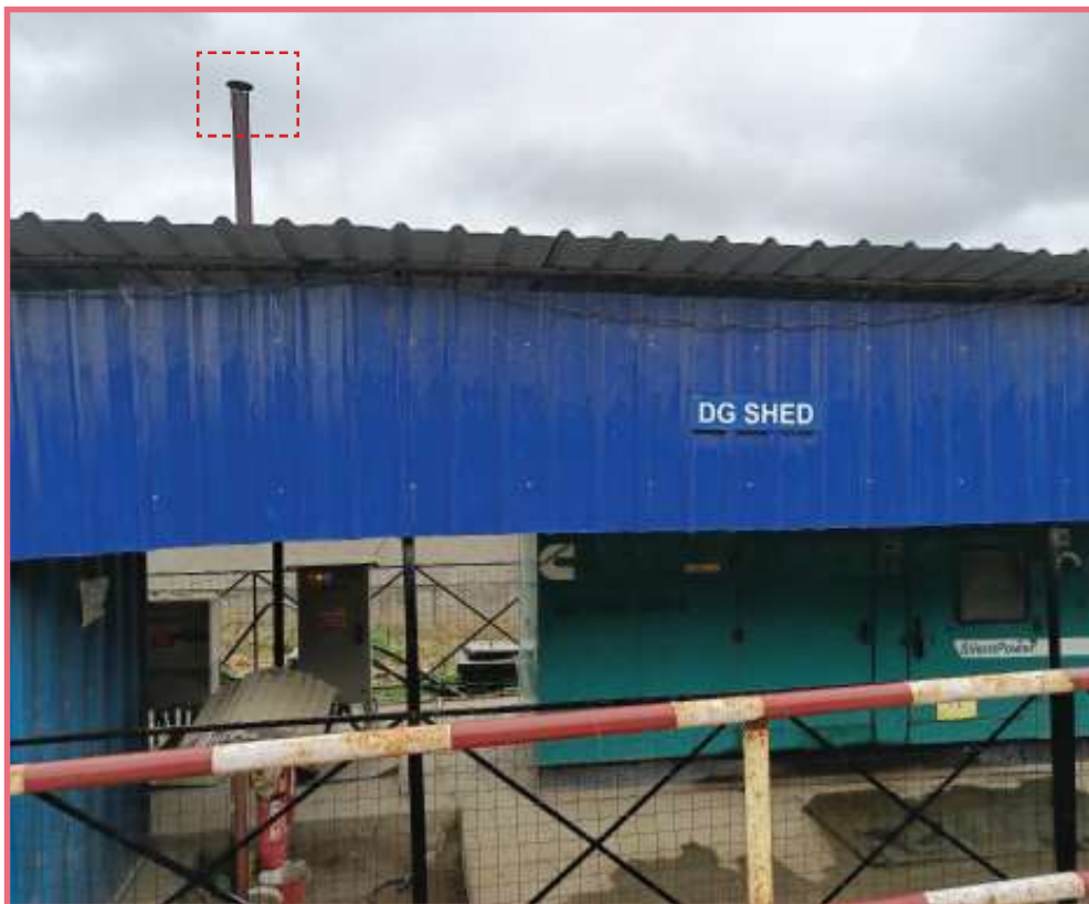
▲ Exhaust (along with a cowl) of a diesel generator with a stack height of 2m from the top of DG set
