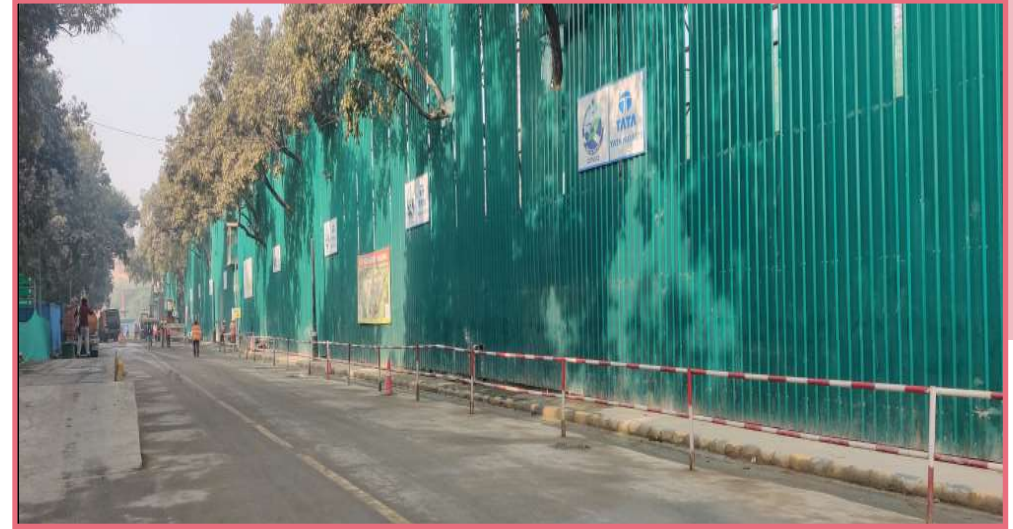
▲ Barricading done by galvanized iron sheets
