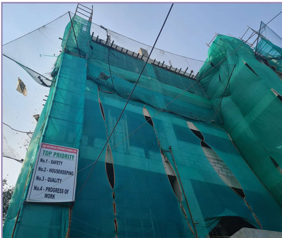
▲ Provision of safety nets at height in a building under construction
