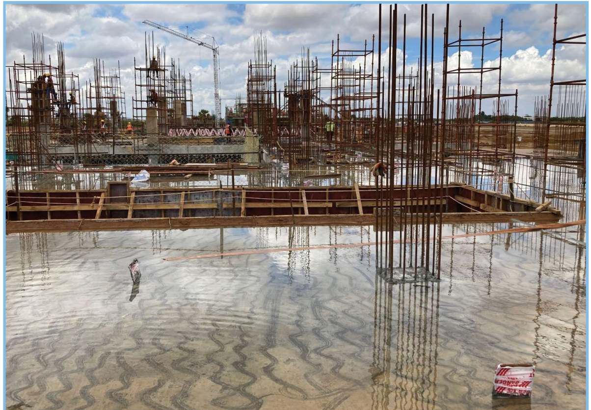
▲ Ponding technique used for curing of concrete
