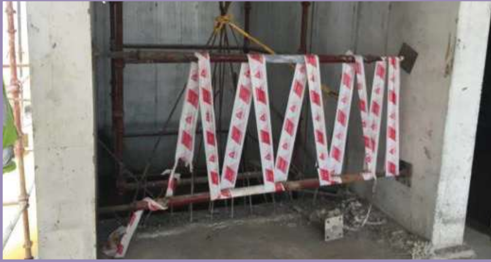
▲ Demonstration of barricading of open lift shafts on-site
