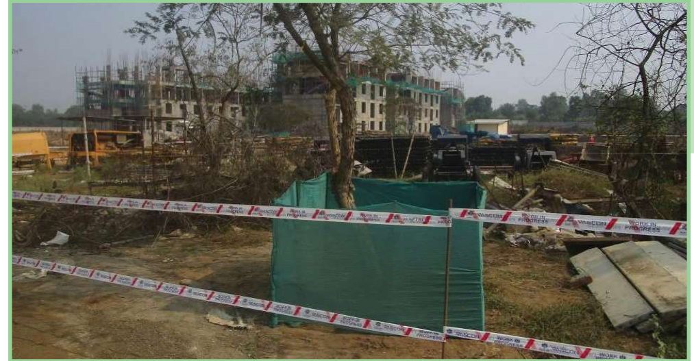
▲ Demonstration of barricading of trees using green net and tape
