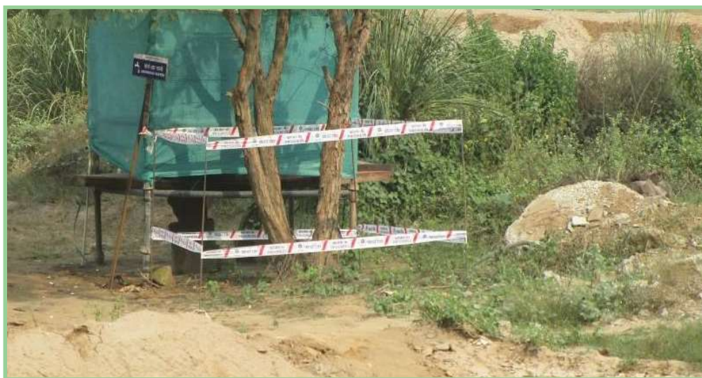
▲ Demonstration of barricading of trees using steel rods and safety tapes
