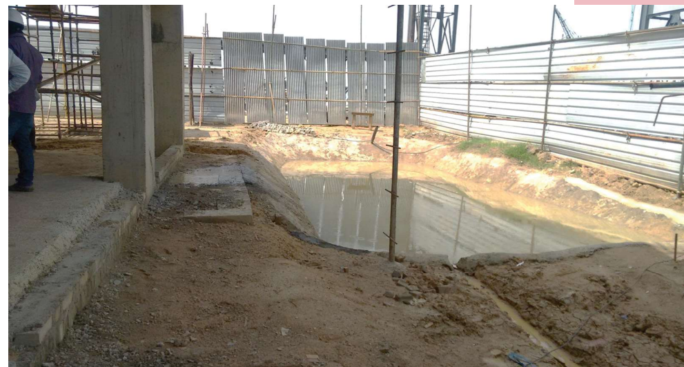
▲ Sedimentation tank connected via soil erosion channel
