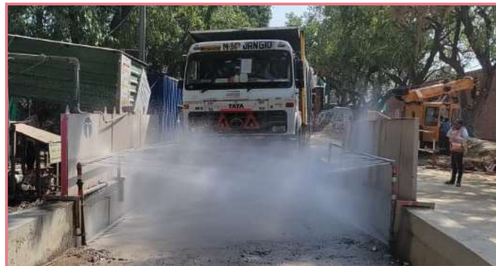
▲ Tyres of a truck getting washed by a mechanical wheel-washing facility
