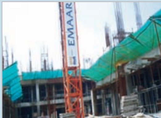
Figure 4 Safety nets at construction site
