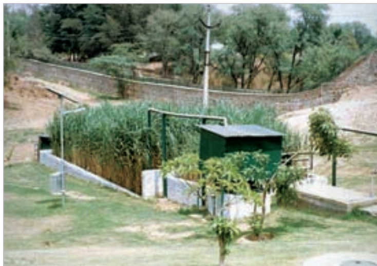
Figure 7 Root zone system for waste water treatment
