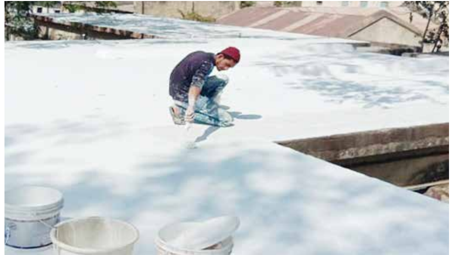
Cool roof paint being applied at Kannad (Credits: Author)
