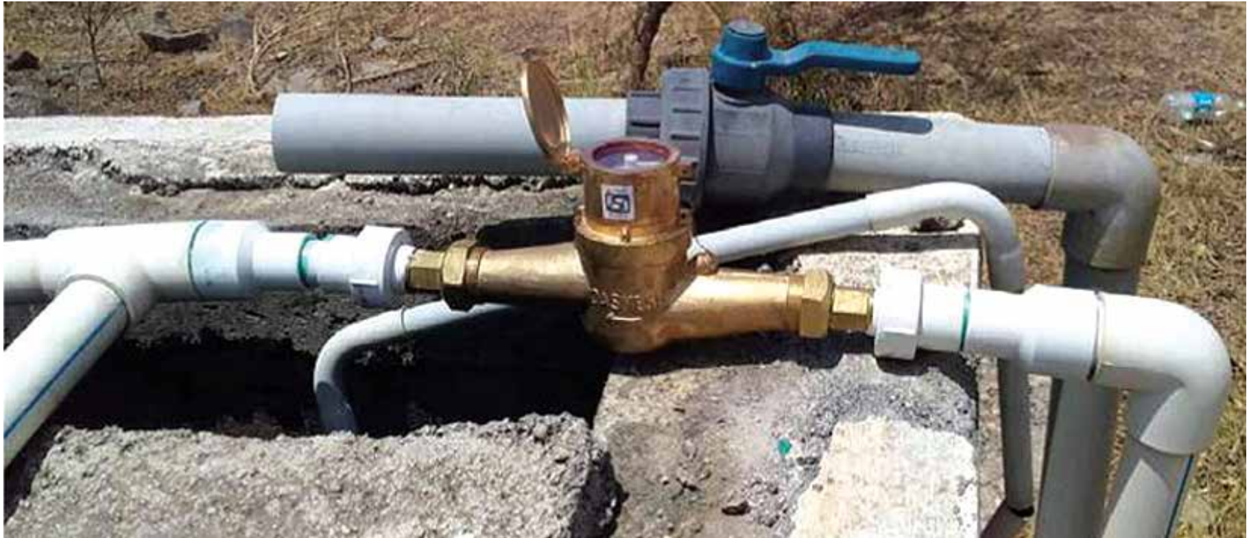
Water meters installed at the hospital (Credits: Author)
