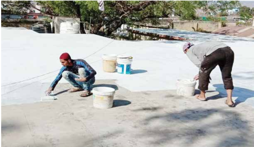
Cool roof paint being applied at Kannad (Credits: Author)
