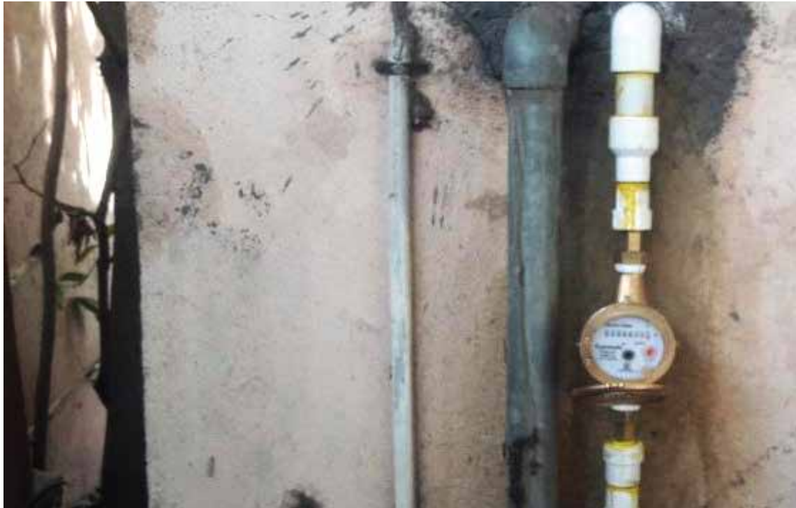
Water meters installed at the Renapur hospital (Credits: Author)
