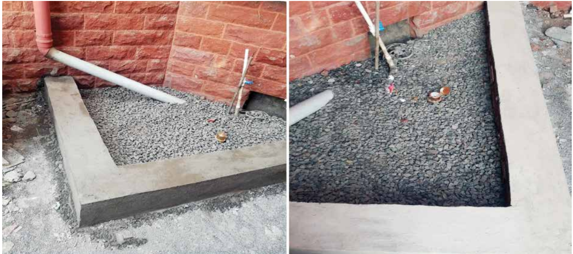
Rainwater harvesting pit with a water meter (Credits: Author)
