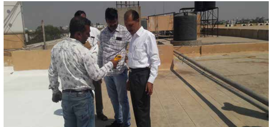
PHOTO 4.4 PWD officer inspecting the application of high SRI paints on roofs
