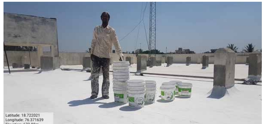
PHOTO 4.5 Roof painted with high SRI paint
