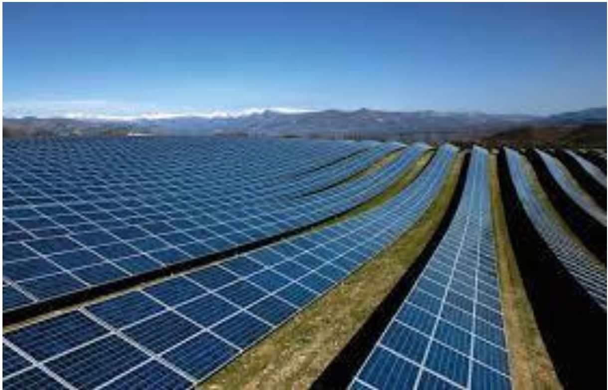
Figure 6.3: Rewa solar power project
