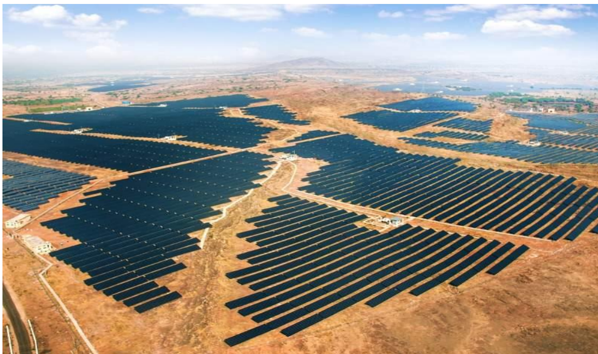
Figure 6.2: Bhadla Solar Park
