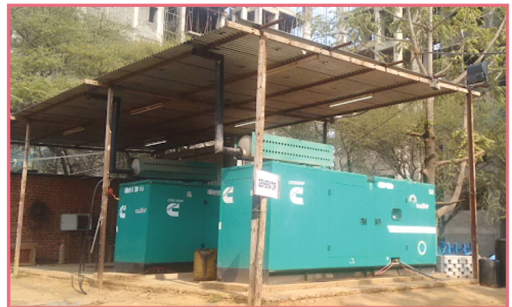
▲ Diesel generator placed on site away from the construction zone
