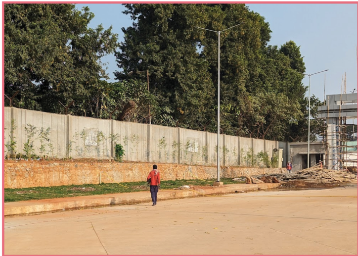
▲ Barricading done by solid concrete wall
