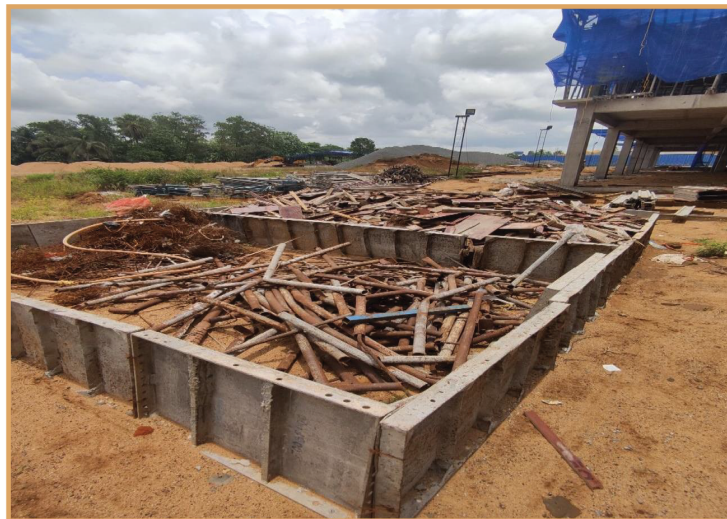
▲ Demonstration of segregation of steel scraps
