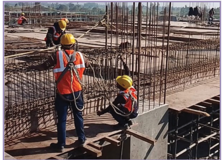
▲ Adherence of workers with safety harnesses working at height on-site.
