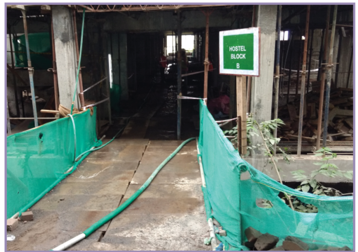
▲ Barricading along the crossway
