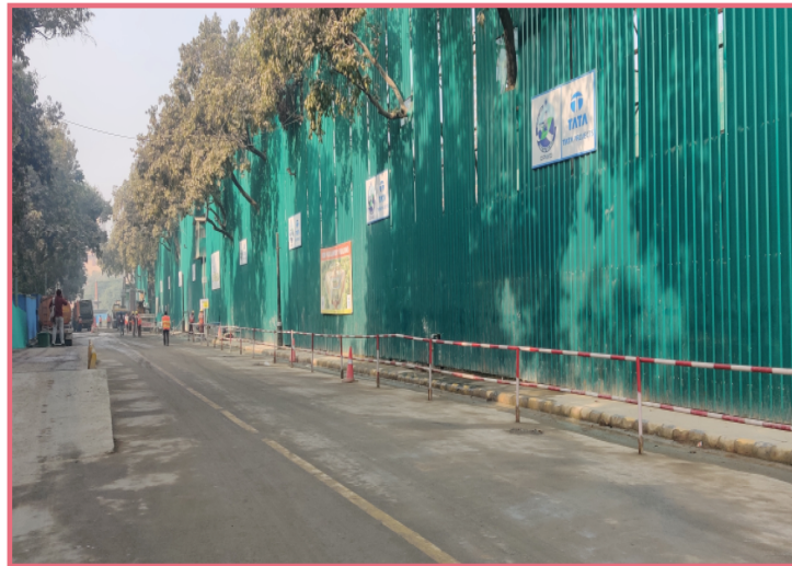
▲ Barricading done by galvanized iron sheets
