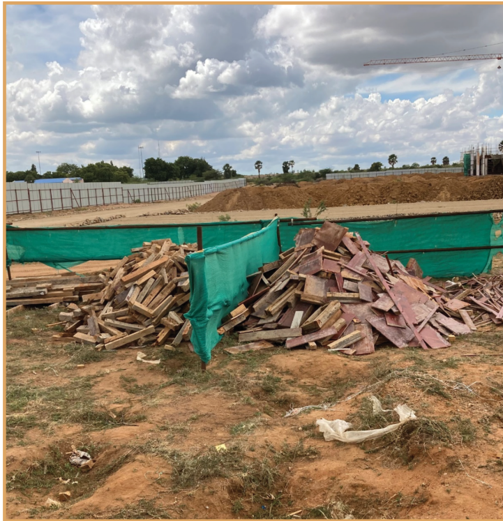
▲ Demonstration of segregation of wood scraps | Project location: Jajpur, Odisha
