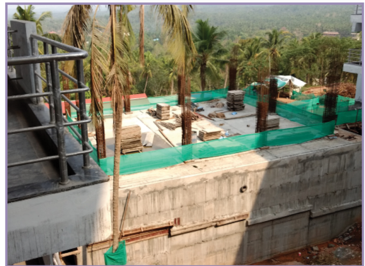
▲ Barricading of open slab on-site
