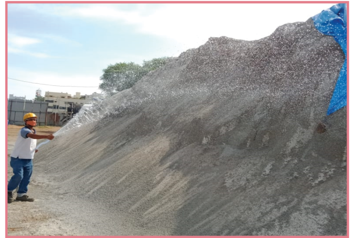
▲ Fine material being sprayed on with water by a worker
