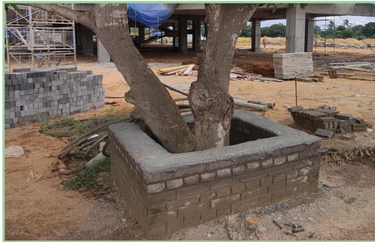
▲ Demonstration of barricading of trees using concrete blocks
