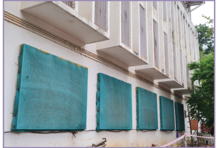
▲ Barricading of openings on the construction site
