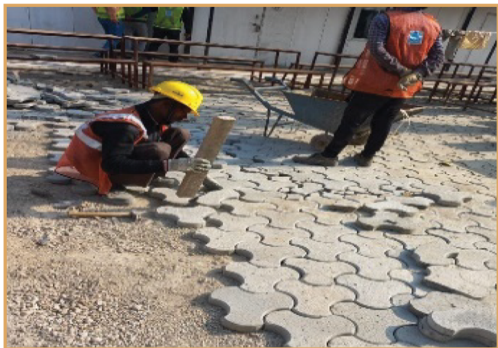
▲ Demonstration of reuse of waste concrete used on site | Project location: New Delhi
