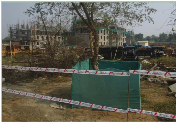
▲ Demonstration of barricading of trees using green net and tape
