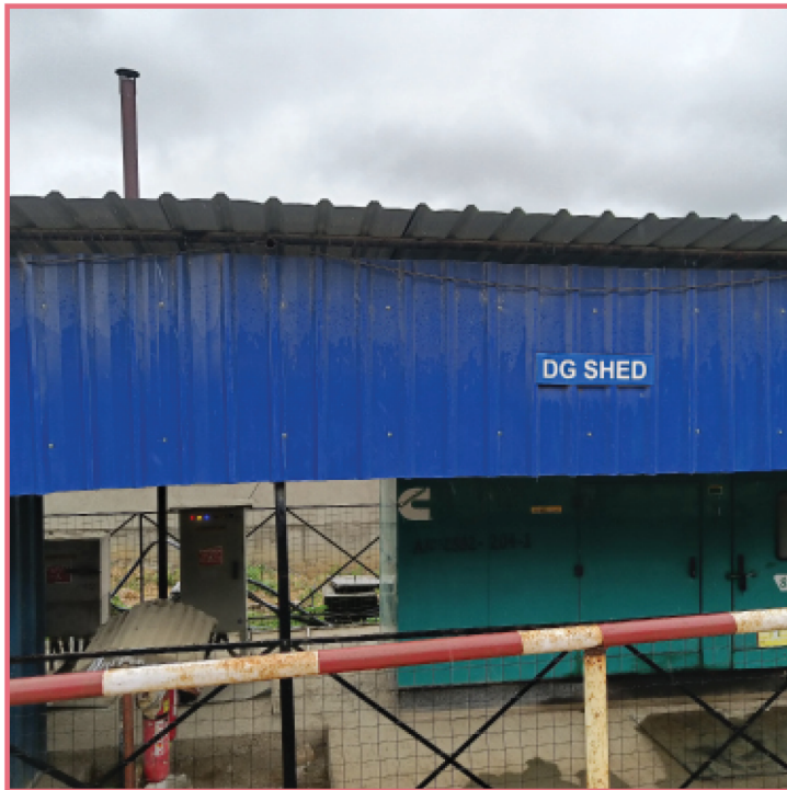
▲ Exhaust (along with a cowi) of a diesel generator with a stack height of 2m from the top of DG set
