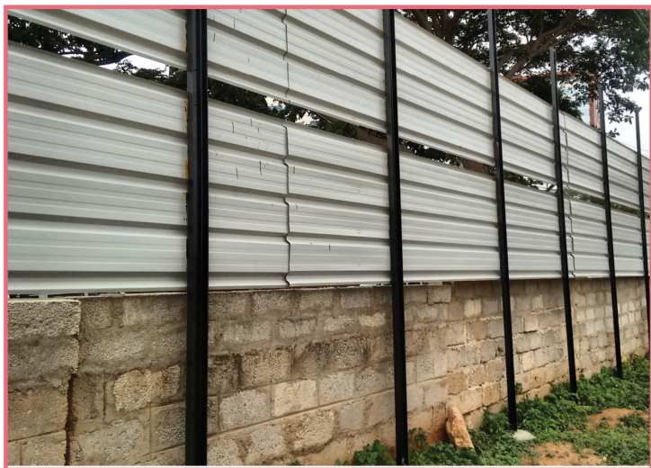
▲ Permanent barricading height increased by adding galvanized iron sheets
