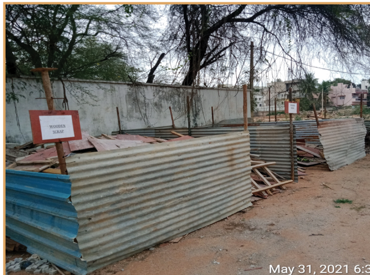
▲ Demonstration of segregation of construction waste
