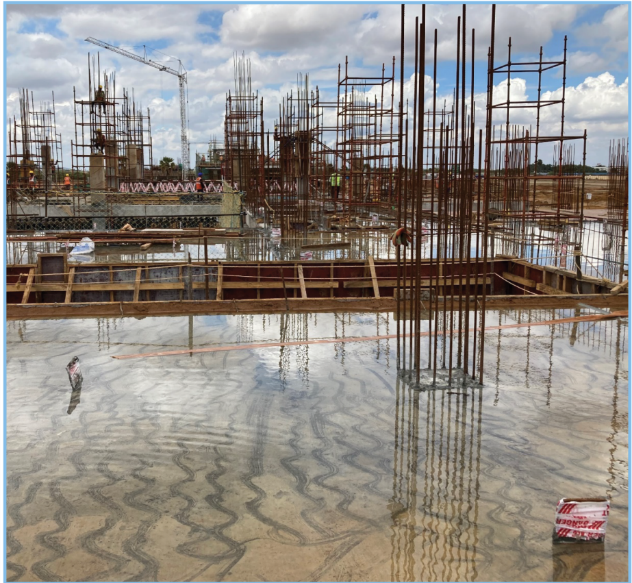
▲ Ponding technique used for curing of concrete
