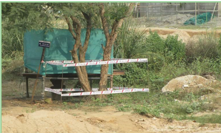
▲ Demonstration of barricading of trees using steel rods and safety tapes
