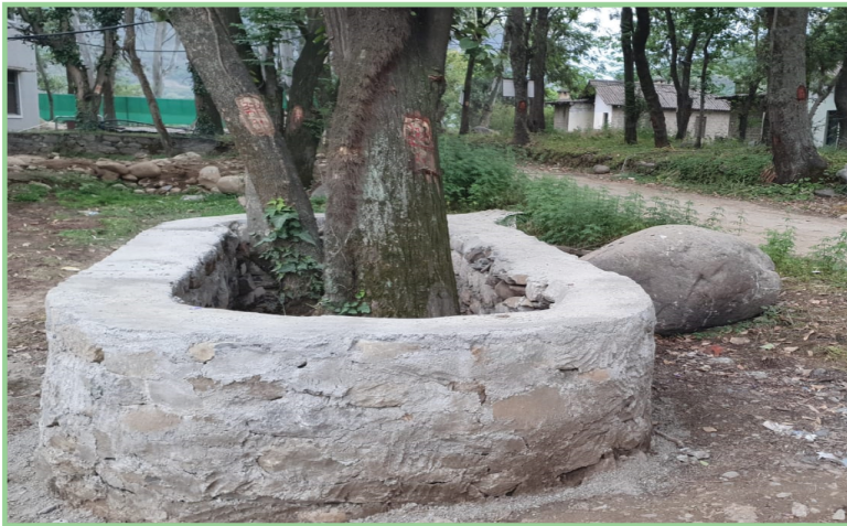
▲ Demonstration of barricading of trees using rubble masonry
