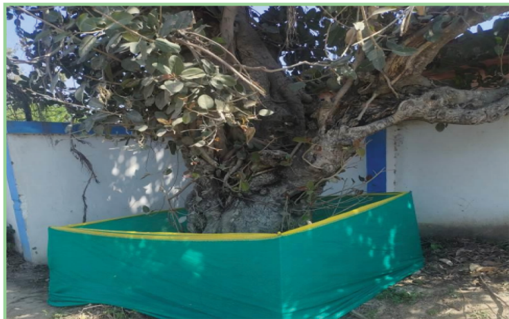
▲ Demonstration of barricading of trees using green net
