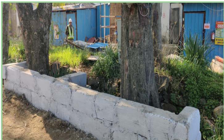
▲ Demonstration of reuse of waste concrete blocks to safeguard trees
