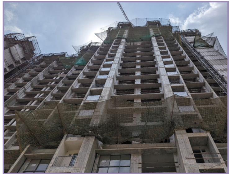
▲ Provision of safety nets for a multi-storey | Project location: Panvel, Maharashtra
