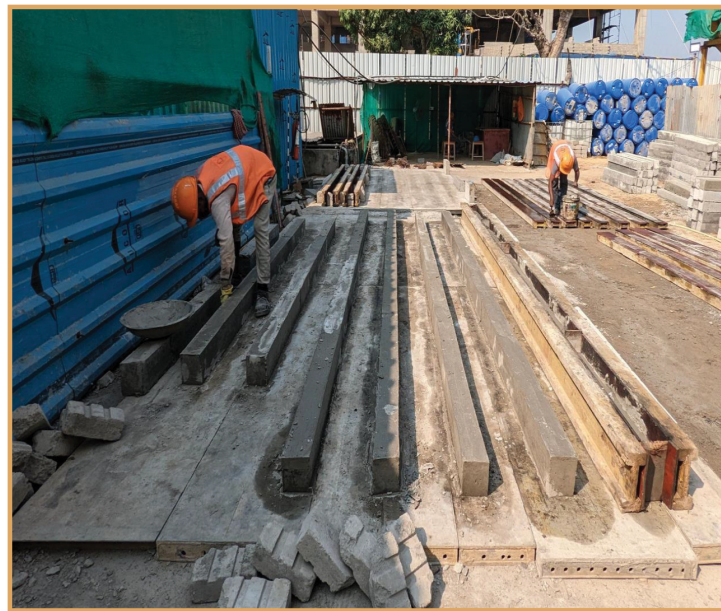
▲ Demonstration of reuse of waste concrete used on site to make lintels | Project location: Jajpur, Odisha
