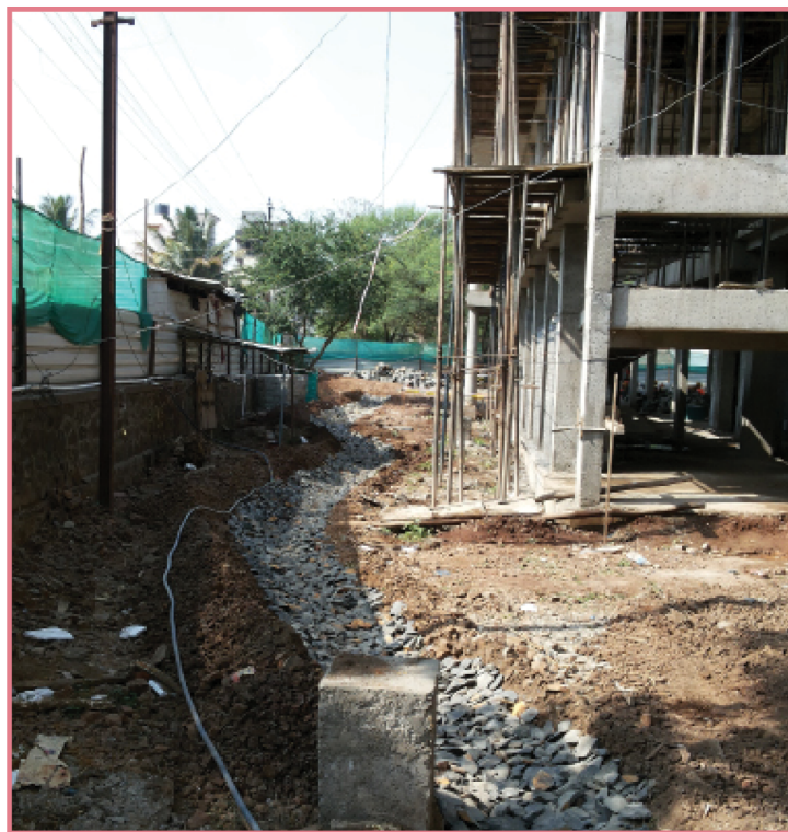
▲ Soil erosion channel with gravel bed
