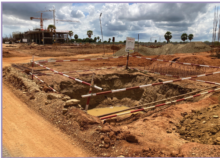
▲ Barricading of excavated area on-site
