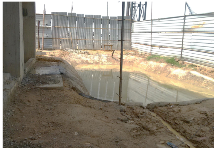
▲ Sedimentation tank connected via soil erosion channel
