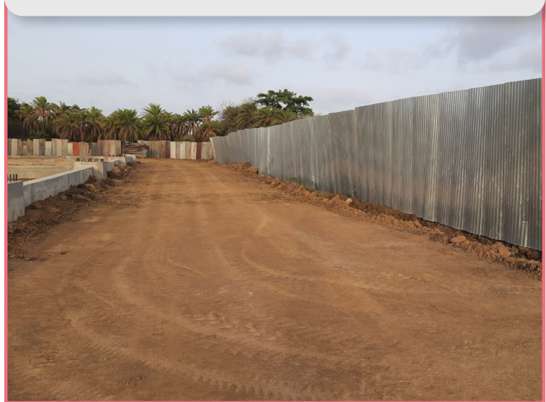
▲ 3 meter high barricading along the site boundary | Project location: Daman
