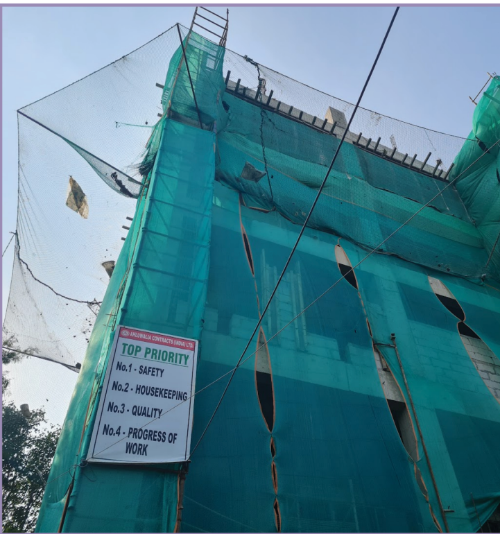
▲ Provision of safety nets at height in a building under construction
