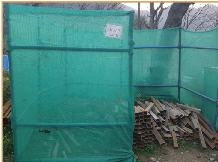
▲ Demonstration of segregation of steel scraps
