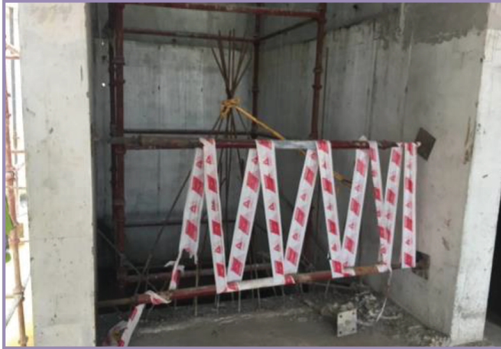
▲ Demonstration of barricading of open lift shafts on-site
