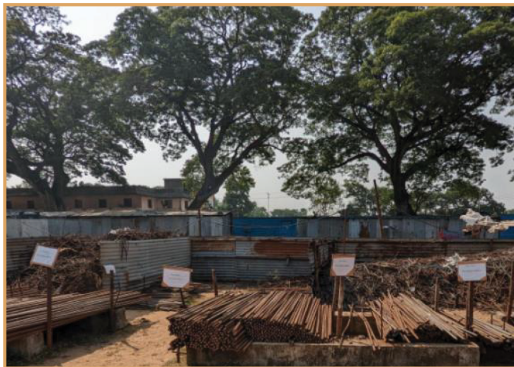
▲ Demonstration of segregation of steel rods of varying diameter
