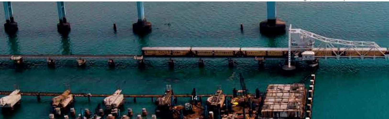
Pamban Bridge, Ramanathapuram
