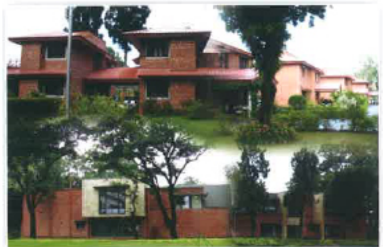
The Doon School: Art School, Main field Master's house (5 numbers) and Hathikhana Master's Houses (5 numbers) - Two Star TERI GRIHA Rated Buildings
